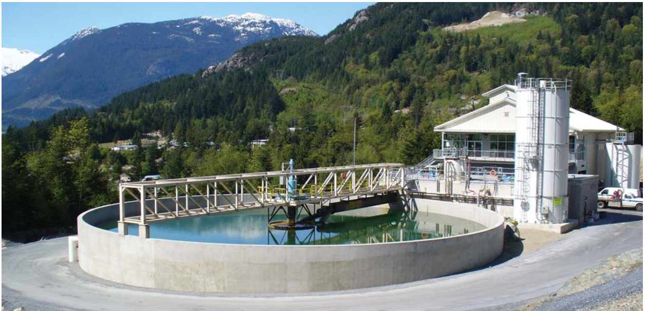
Above Water Treatment plant
